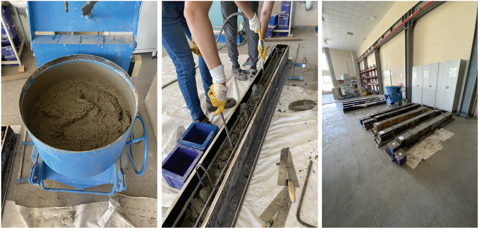
Figure 2 - Steps of concrete pouring
