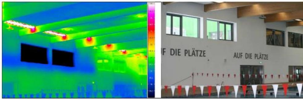
**Figure 7.** Thermal Bridges in Bambados Indoor Pool
