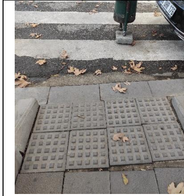
Figure 4. Sensible surface on ramp (A50, A127)
