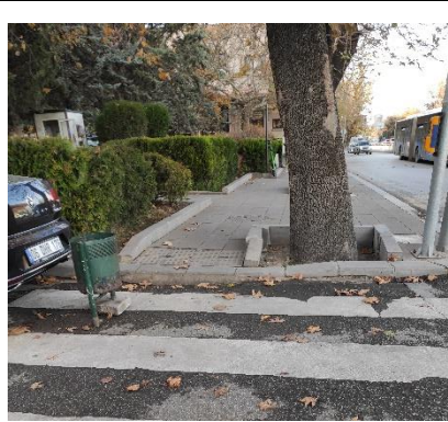
Figure 1. Sidewalk-crosswalk (A50, A128, A131)
