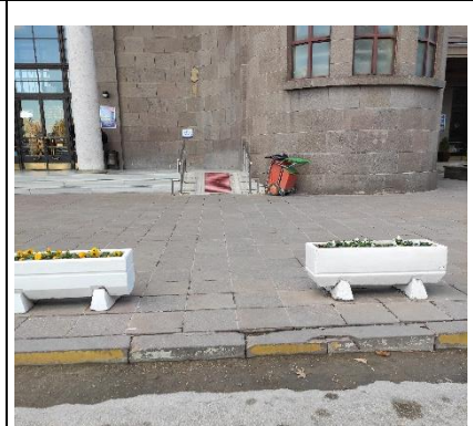
Figure 3. Ramp-stairs (A.6, A50, A56, A57, A88)
