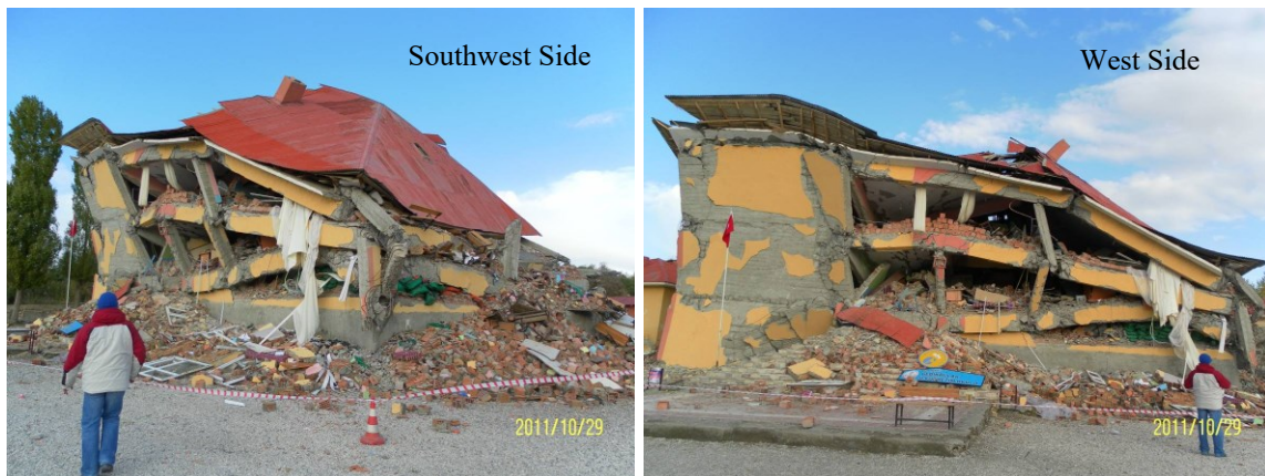
Figure 3. Southwest and west side views of the building.
