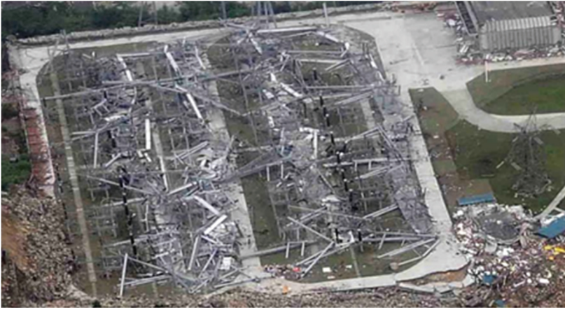
Figure 2 - Ertai Shan Switchyard which had experienced total collapse during the Wenchuan China (2008) earthquake [3]
