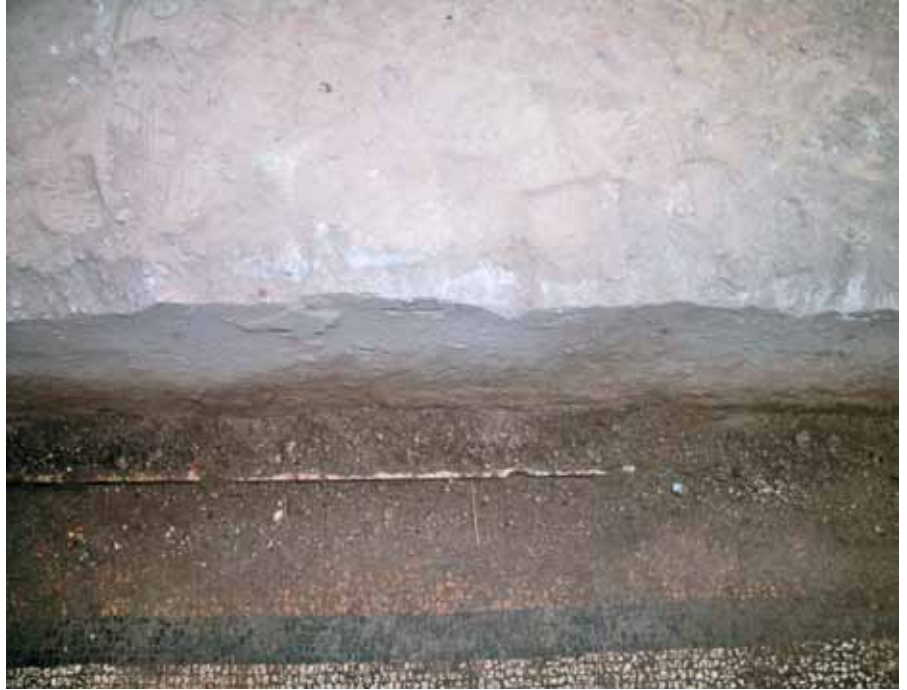
Figure 3 The tibuli system built in front of the wall
