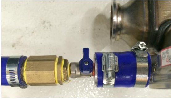
Figure 20. Initial Leak Check Setup
