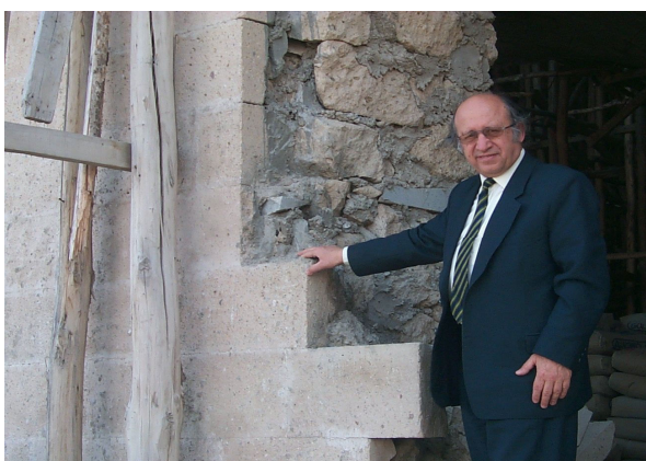
Figure 1. Cladding walls of a mosque with tuffstone in Isparta city
