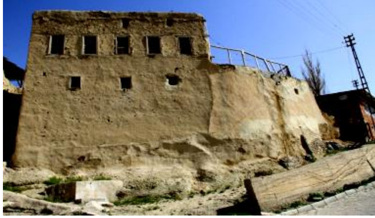
Foto 1b. Güney cephe (Photo 1b. South front)
