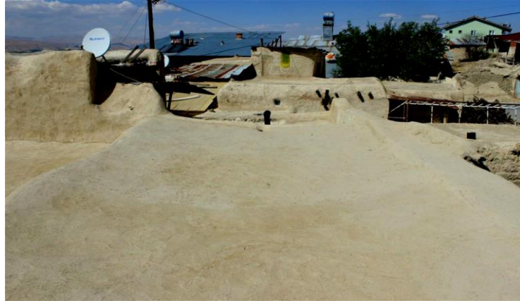
Foto 2j. Toprak dam (Photo 2j. Soil roof)
