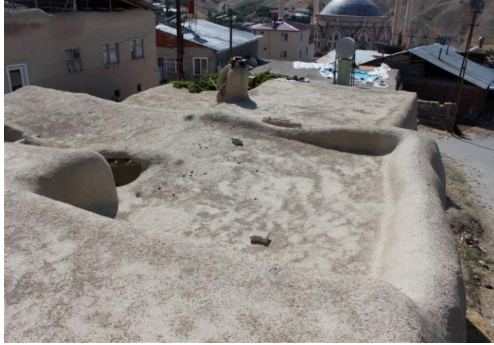
Foto 3h. Toprak dam (Photo 3h. Soil roof)
