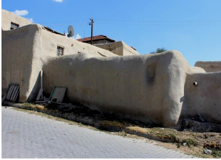
Foto 3d. Kuzeybatı cephe (Photo 3d. Northwest front)
