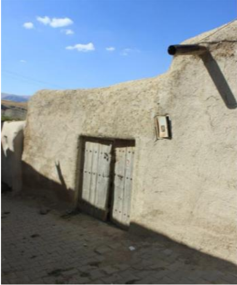
Foto 3b. Güneybatı cephe (Photo 3b. Southwest front)
