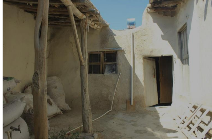
Foto 3e. Avlu kuzey cephe (Photo 3e. Courtyard the north front)
