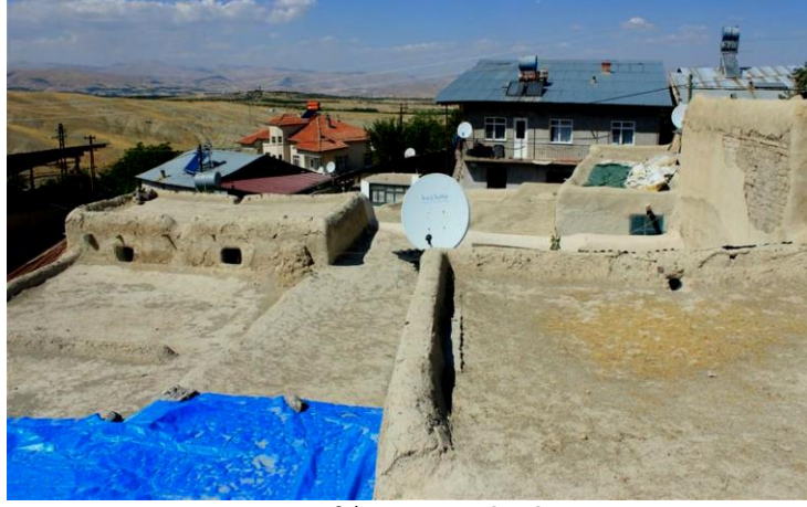
Foto 2i. Toprak dam (Photo 2i. Soil roof)
