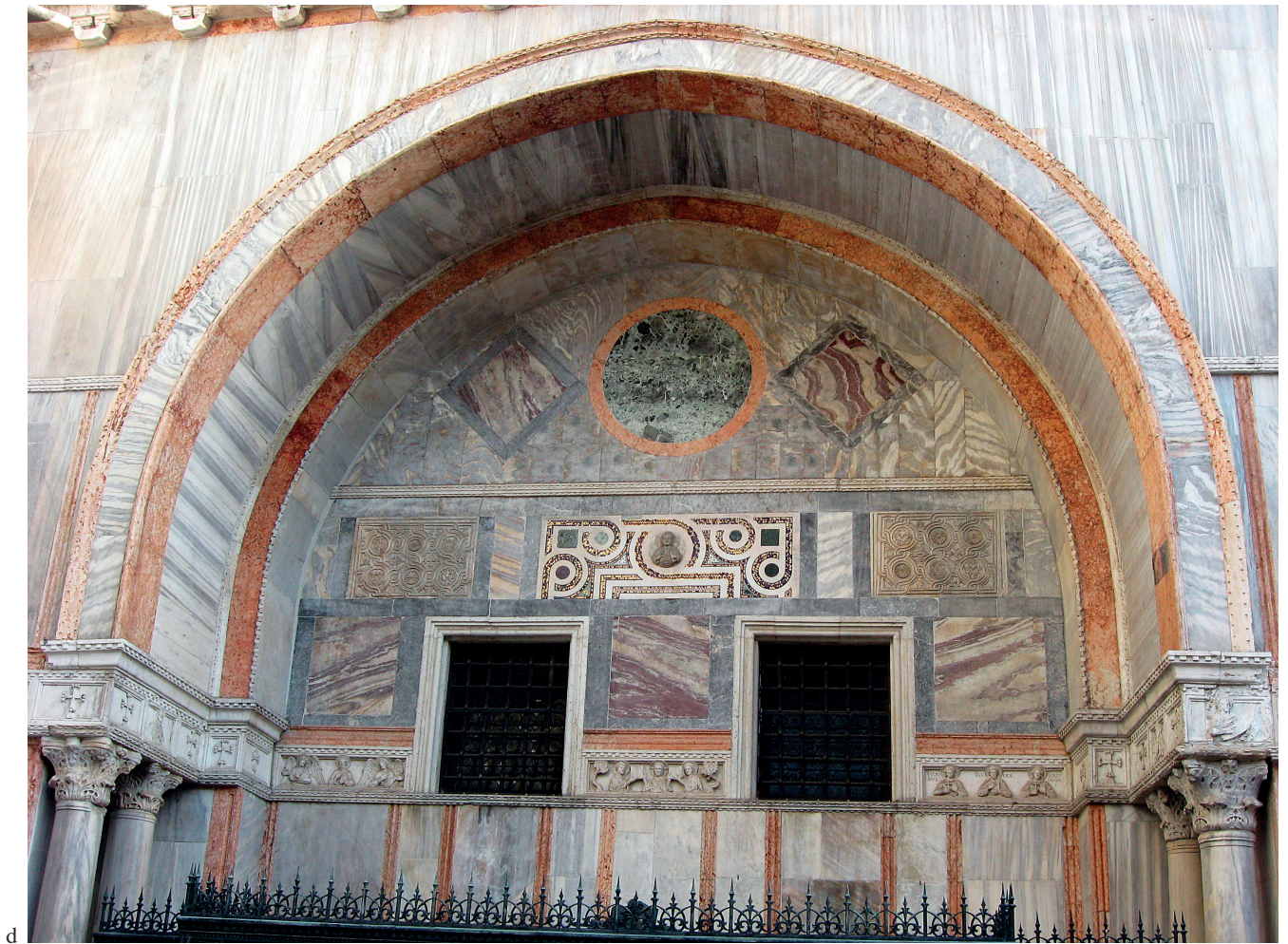
Figure 16 d Photograph. Showing the variety of decorative covering panels from the side entrance of St Mark's Basilica, in Venice Two kinds of fossil-bearing limestone used as ornamental stone for the floors of the inside of this mediaeval monument have been identified. They are from Asia Minor with roots in the tradition of using material from quarries that were exploited in the Roman era (Vio 2012: 83, Lumachela da Megalodon – bivalve Megalodon sp.; p. 87, Occhio di pavone – bivalve, order Rudista). Author: Miguel Pessoa. 2013
