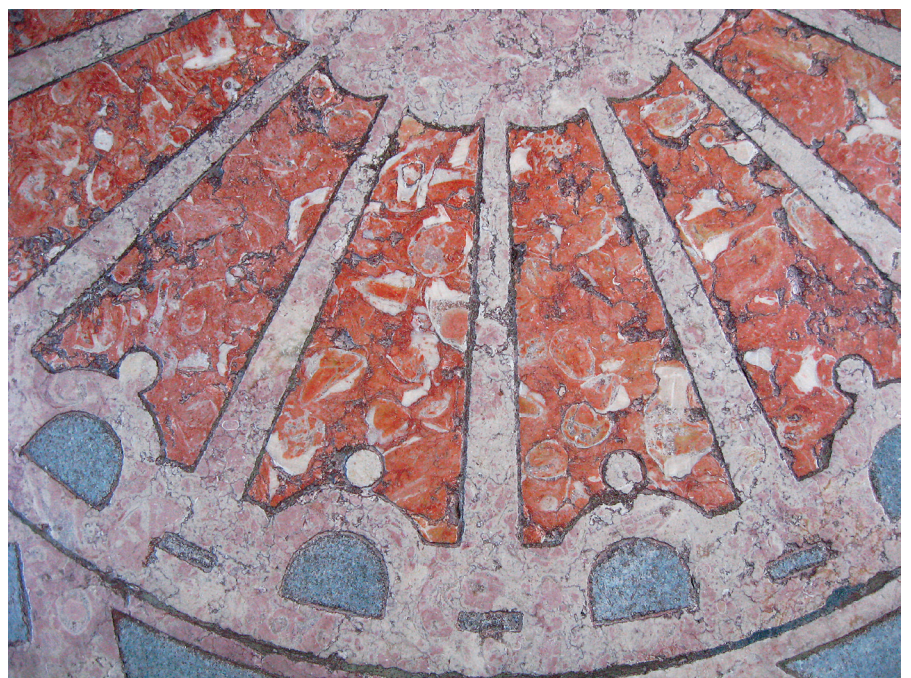
Figure 16 e Photograph. Detail of polished rudist limestone or lioz limestone panels. Polychrome inlays, using various kinds of cretaceous limestone, and the blue limestone from Sintra. Background shaded with yellow and red. Preserved in situ in the floor of the corridor on the west side of the 1 st floor of the National Palace of Mafra. It resembles the one preserved in the floors of the Estrela Basilica (Aires-Barros 2001: Vol. I 93, Photo 29). Author: Miguel Pessoa. 2013
