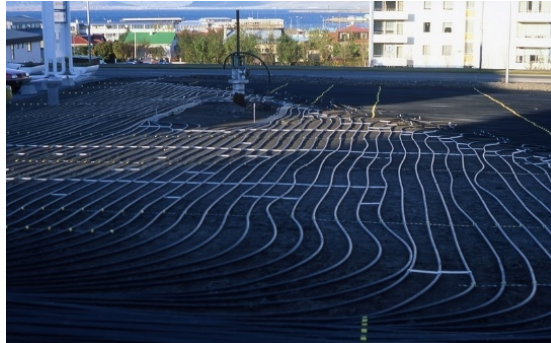
Figure 5. Melting snow and preventing ice conditions on the road by geothermal energy
