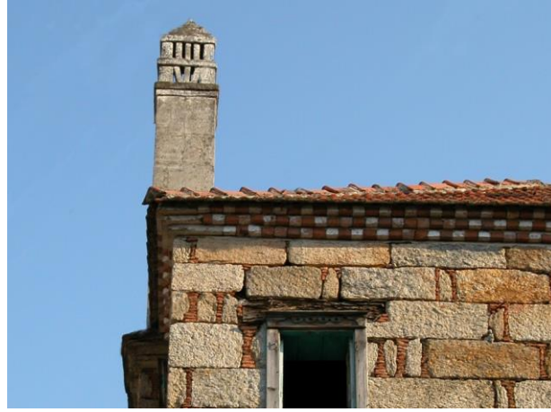
Figure 18. Original cornices of Çomakdağ houses made with three rows of bricks. (photo belongs to the author)
