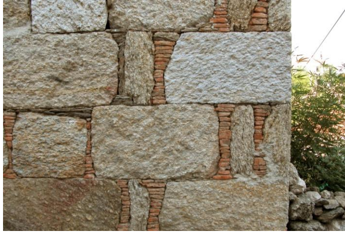
Figure 11. Details from stone masonry whith joints between the stones are tightened with 15-20 cm. long, 5-8 cm. wide pieces made of crushed olive oil potteries called nails Çomakdağ / Kızılağaç house (photo belongs to the author)
