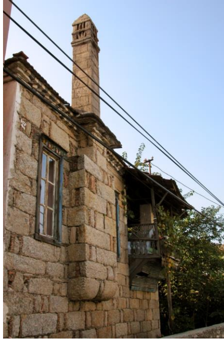
Figure 14. Typical chimney form which projects from the facade (photo belongs to the author)
