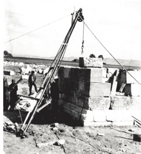
Fig. 4) Mausoleum under works of reassemble in 1967 (Vérité 1988)
