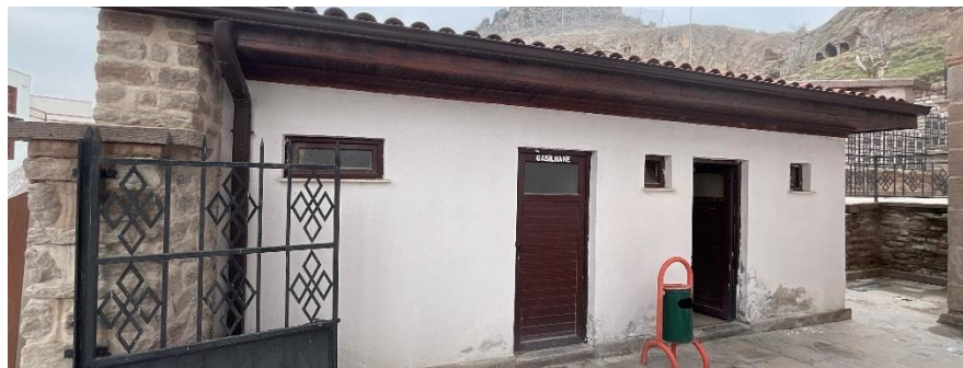
Figure 17. The view of the structure consisting of a funeral washing room, ablution area, toilet, and washbasin
