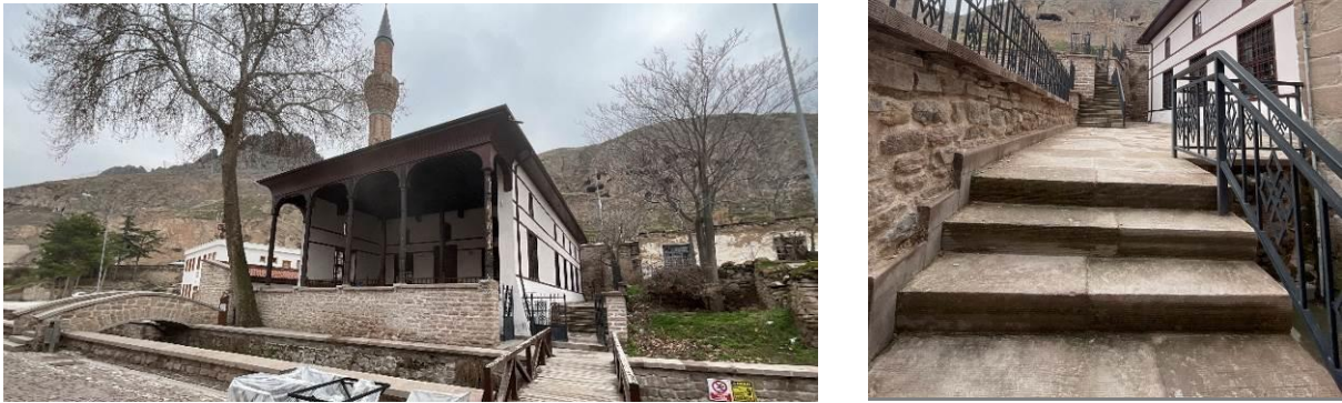
a b Figure 4a-b. Connections of Sille Çay Mosque with the streets
