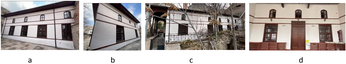
Figure 9a-b-c-d. The view of the facade views of Sille Çay Mosque
