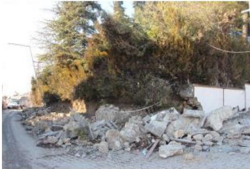
Figure 31. The slid pavement due to lateral movement of retaining wall
