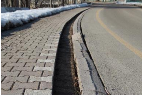
Figure 31. The slid pavement due to lateral movement of retaining wall
