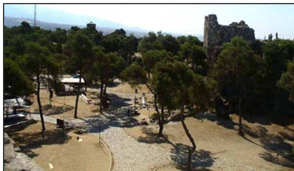
Figure 2. General view of Kadifekale.
