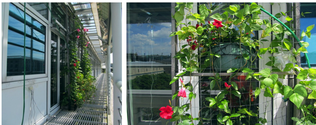
Figure 16. PM_{2.5} sensors @ control façade.
