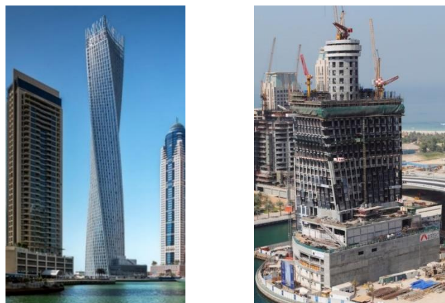
Figure 9. View of Cayan Tower [24] and construction progress [25]
