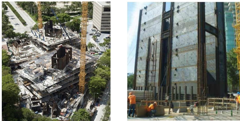
Figure 7. Aerial view of composite shear walls and steel plates within composite core [23]
