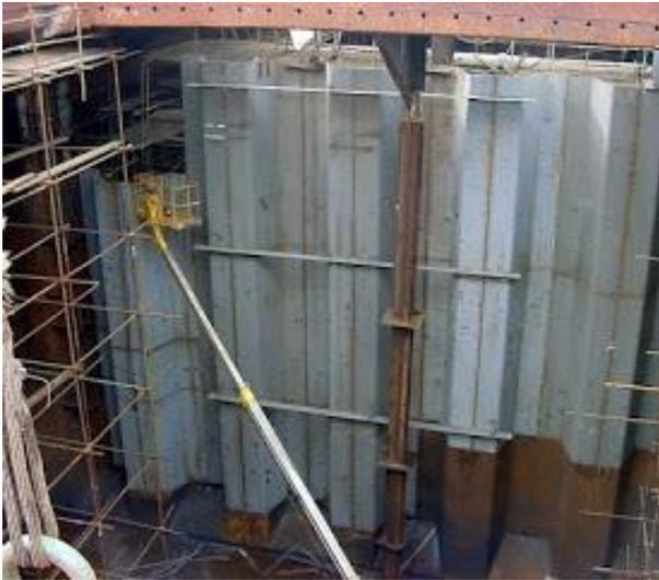
**Figure 1.** A typical corrugated bulkhead structure shown
