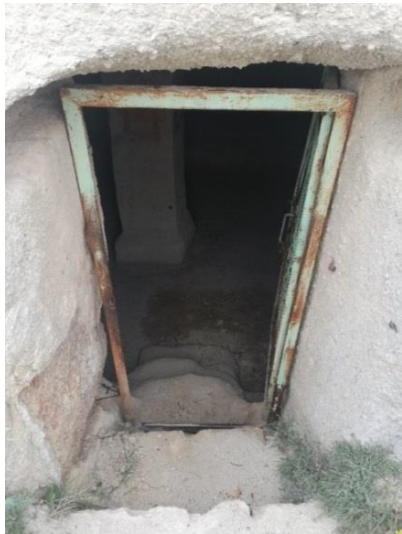
Figure 14. The Saklı Church entry door distortion detail (Ertürk, 2020, p.145)
