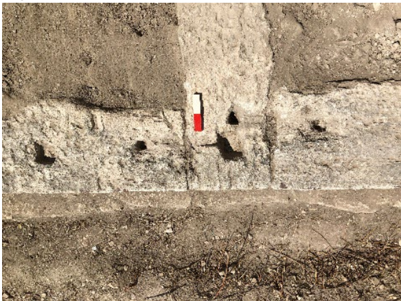
Figure 19 Clamp slots in balustrade
