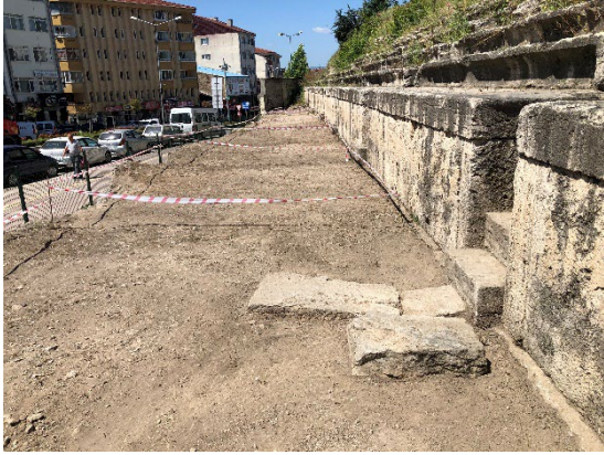
Figure 9 Work on the trenches in front of the Stadium
