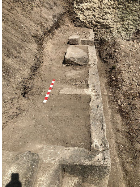
Figure 18 Internal view of the balustrade
