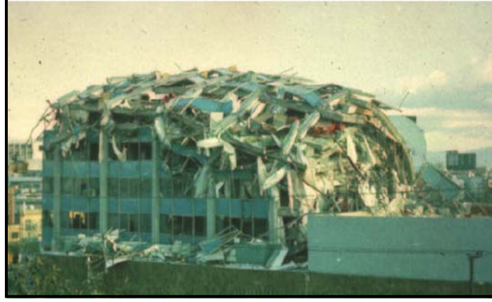
Şekil 3. 1985 Meksika depreminde hasar görmüş bir bina (Güney, 2015) Figure 3. A damaged building in 1985 Mexico City earthquake (Güney, 2015)
