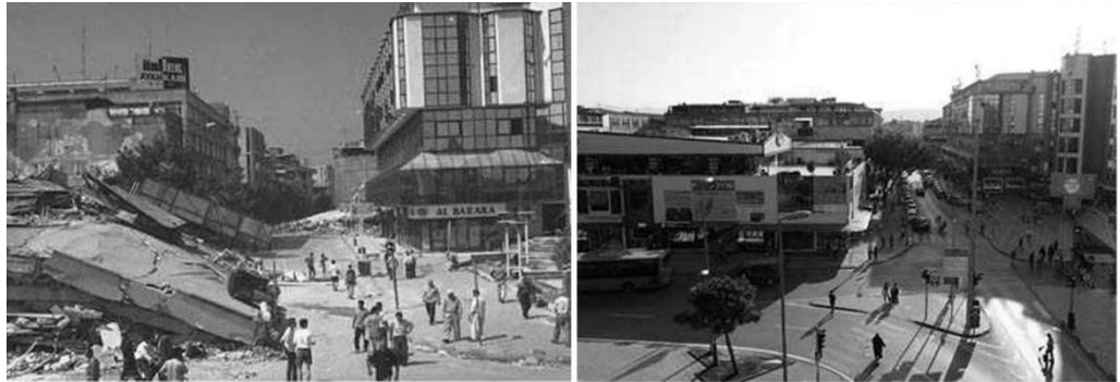
Figure 20. The view of Çark Street in the Adapazarı district of Sakarya, damaged in the 1999 Marmara earthquake, 20 years after the earthquake (Mediabar News Archive, 2019).
