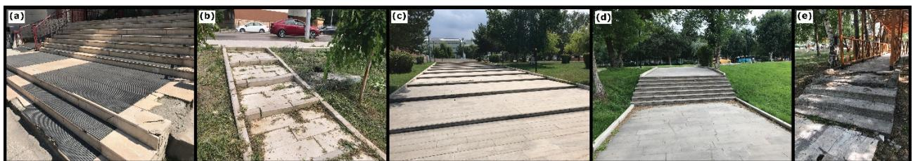
**Figure 5. Stairs-marble Stone (a), Stairs-Andesite Stone (b,c,d), Stairs-Concrete (e)**
