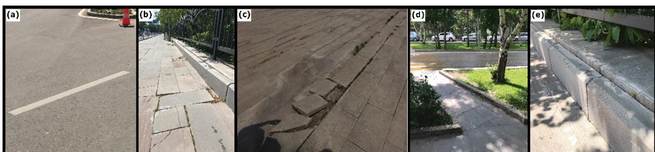
**Figure 2. Vehicle Road-Ashphalt (a), Pedestrian Crossing-Concrete Slab (b,d), Pavement-Concrete Slab (c), and Curb-Concrete (e)**
