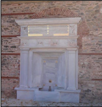
Figure 3. The fountain situated on the exterior garden wall of Beylerbeyi Palace (Original, 2013)
