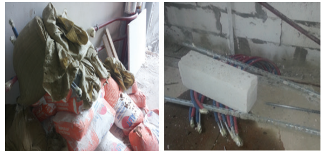
Figure 5. Application example of construction system fault (B3).
