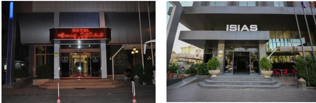
Figure 6. a-b. Hotel entrance after extensive- major renovation (GIO, 2023)
