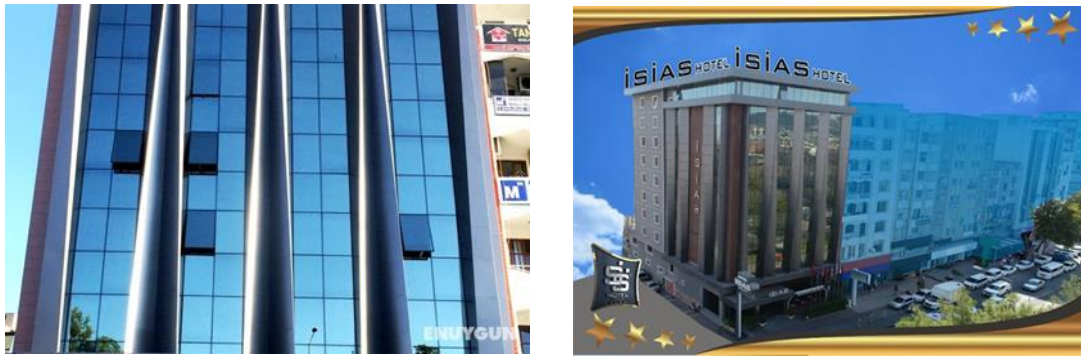
Figure 15.a-b. Exterior image of the hotel after renovation (GIO, 2023).
