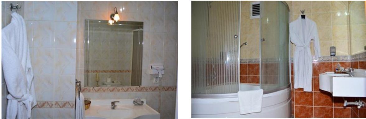
Figure 12.a-b. Pictures from the hotel bathrooms before the extensive-major renovation (GIO, 2023).
