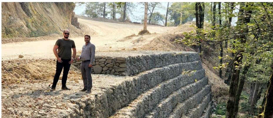
Figure 31. Km: 4+950 after construction and backfill
