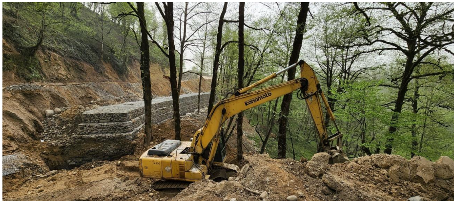
Figure 30. Km: 4+950 during construction
