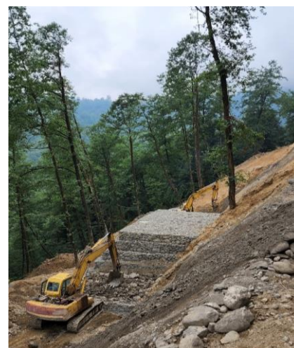
Figure 26. Gabion retaining wall km:3+200.
