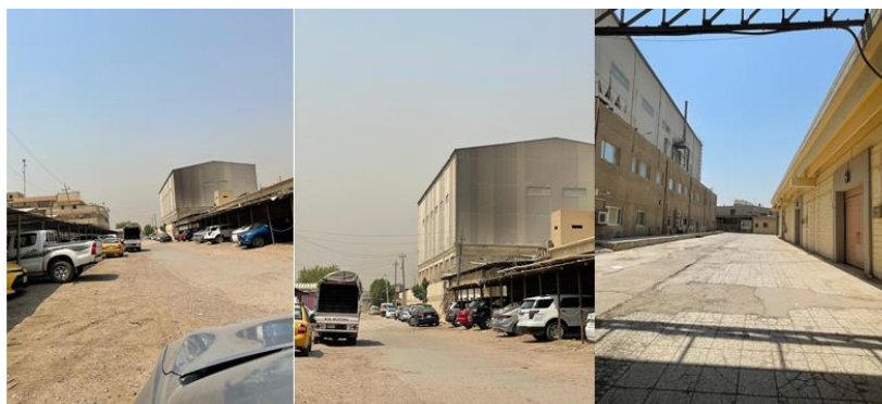
Figure 1. Selected Building (Printing House Al Sabah Newspaper).
