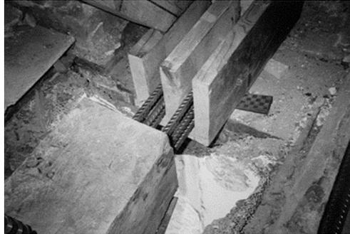
**Figure 11.** The decayed beam end is removed, and the prefabricated softwood replacement beam end is nearly in position. Reinforcement bars are placed in holes drilled in the existing oak [21].
