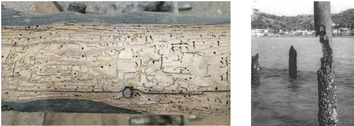
**Figure 1.** (a) Flight holes created by insects at the wooden beam; (b) Port Moresby, Papua New Guinea: CCA-treated hoop pine pilings destroyed by infestation in the intertidal zone by *Sphaeroma triste* [11].
