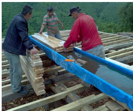
**Figure 3.** The procedure of impregnation done on new wooden elements to be used for restoration[20].
