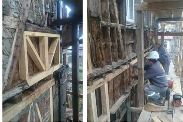
**Figure 7.** Partial replacement in the historical and traditional wooden carcass wall system [25]
