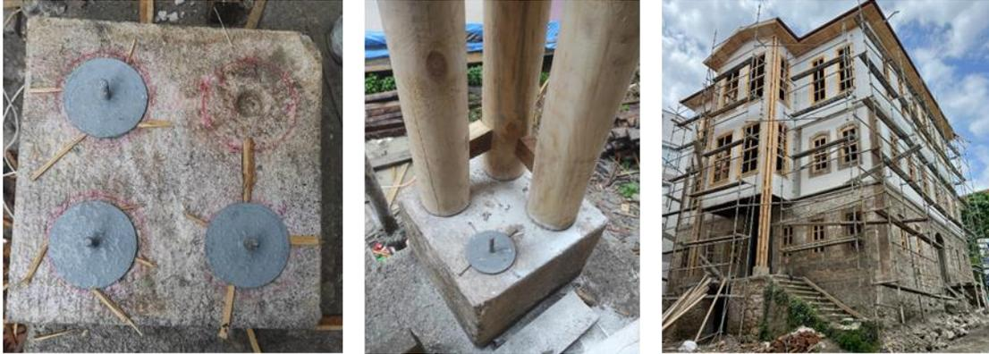
**Figure 5.** Complete replacement on the historical wooden stud; from left to right: fixing metal plates to the rock, fixing new wooden studs to the metal plate, view of wooden studs from the frontal facade [23].
