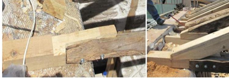
**Figure 9.** Prosthesis application with steel screws [30]
