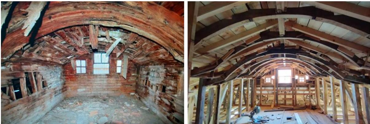
*Figure 4. Complete replacement on the historical wooden roof that is still being restored [23].*
