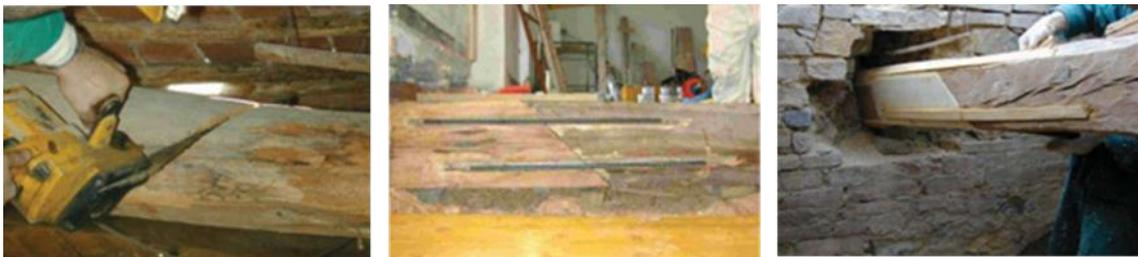
**Figure 12.** The beam end prosthesisation effort made with FRP rods are performed in the following order: inclined cut of decayed end, linking grooves and insertion of a final wedge [31]
