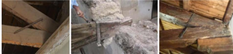
**Figure 10.** Prosthesis application with traditional steel straps [30].
