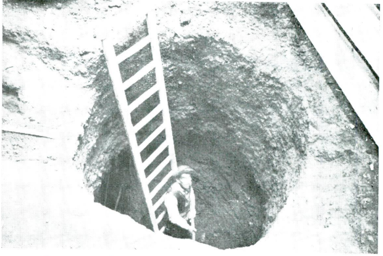
Res. 11 — Daha su çıkmadan kuyudan bir görünüş. Fig. 11 — A view of the well before the level of water was reached.
