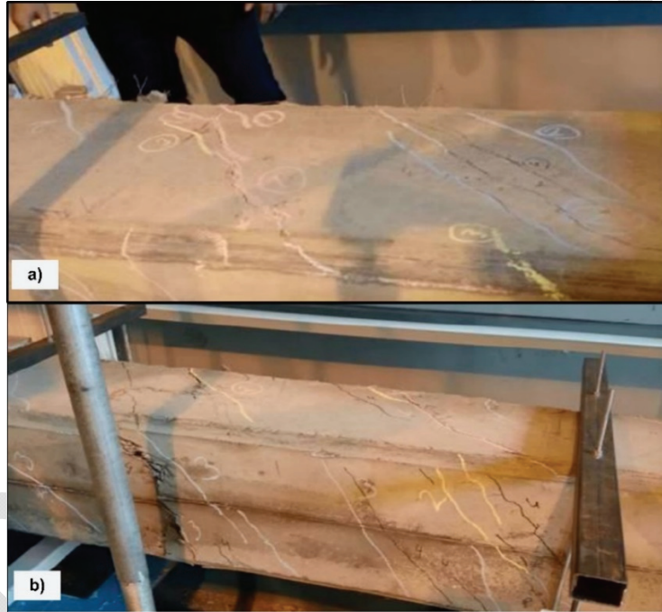
Figure 9 - Crack pattern of S30V15 (a) and S40V12 (b) beams
