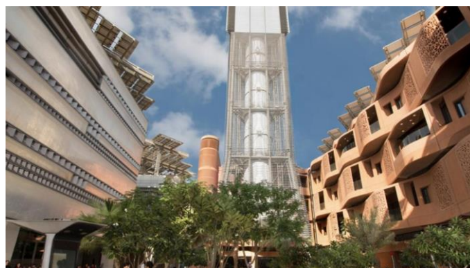
Figure 9. Masdar city wind tower Source: Cugurullo, 2013
