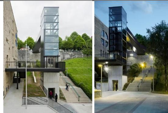
**Figure 20.** Elevator using Hernani, glass and composite coating (MA, EQ) [24]
