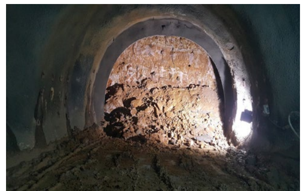
Figure 4. Excavation surface and lining of surrounding rock.
