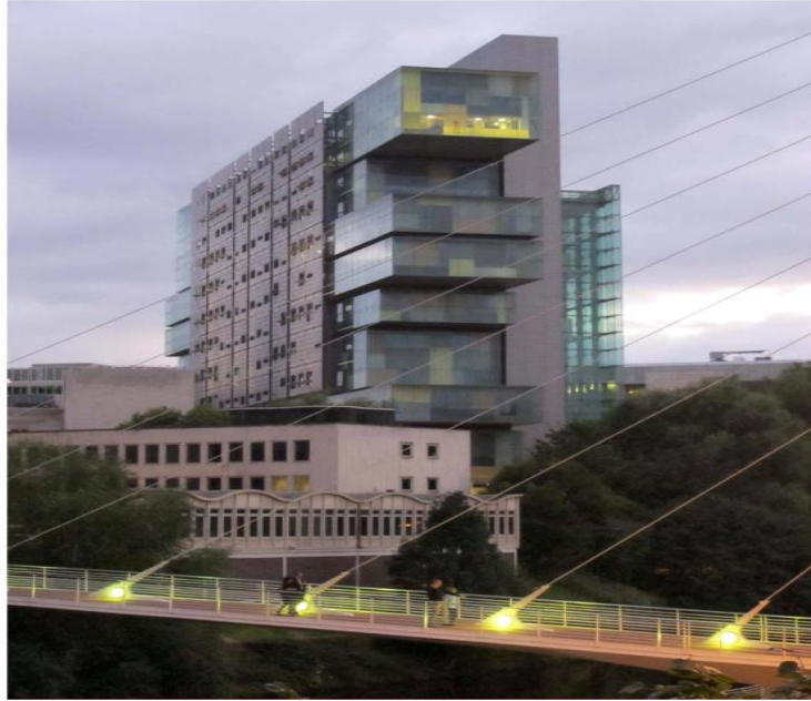
Figure 10. Manchester Civil Justice Centre (Napier, 2013)
