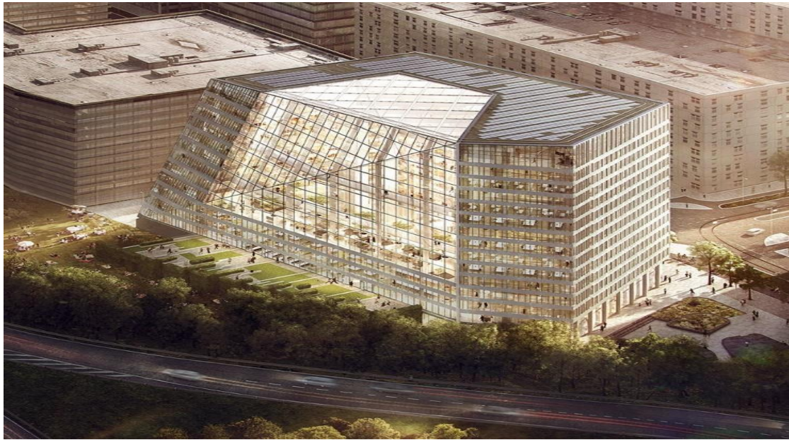
Figure 4. The Edge, Amsterdam. (Jalia and Ramage ,2016)
