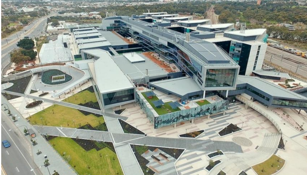
Figure 6. The Royal Adelaide Hospital in South Australia (Sexton, 2017)
