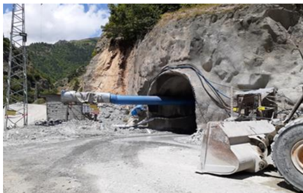
Photo 1. Damla HEPP and Regulator I construction area in Barhal Valley (27.07.2022)
