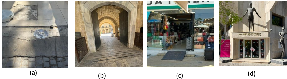
Figure 8. a. Undulated Pattern of the Entranceway, b. Slippery Surface of Great Inn Building Entrance, c. Portable Ramp at Shop Entrance, and d. City Museum Entrance with Leveled Surface is not Appropriate for All Seniors (Güvenbaş,2023)
