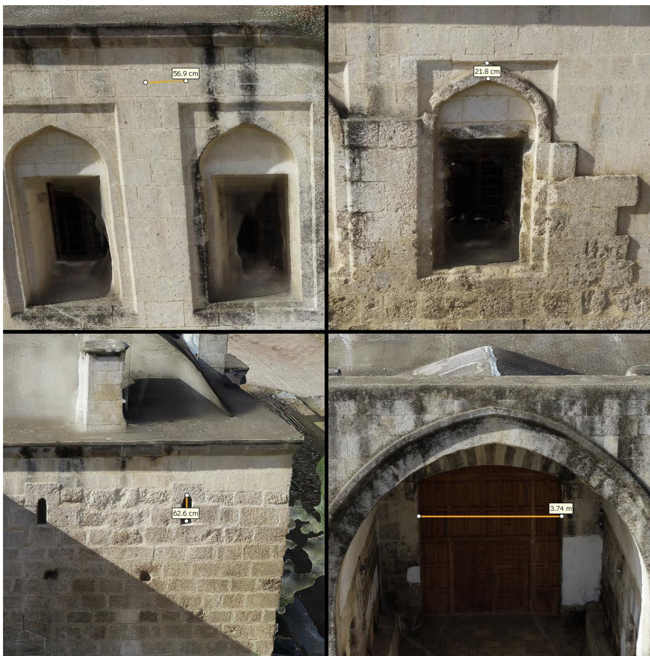
Figure 10. The metric information of some building elements taken from the 3D model of the caravanserai.
