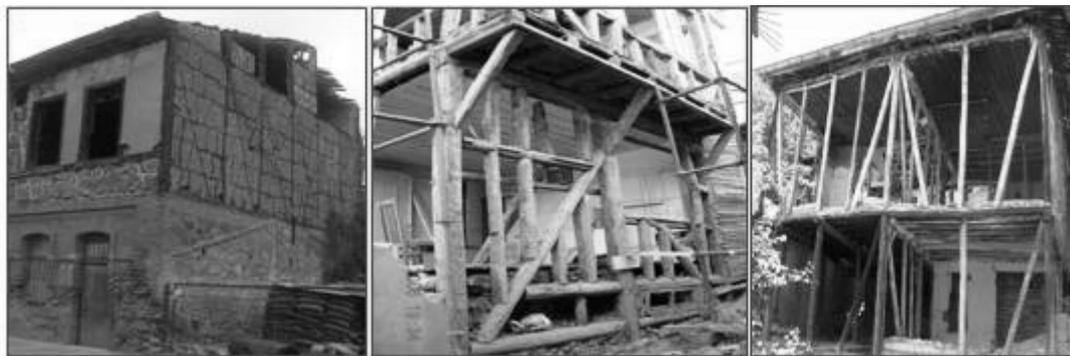
Figure 11. Wooden bearing system and its overhangs.
