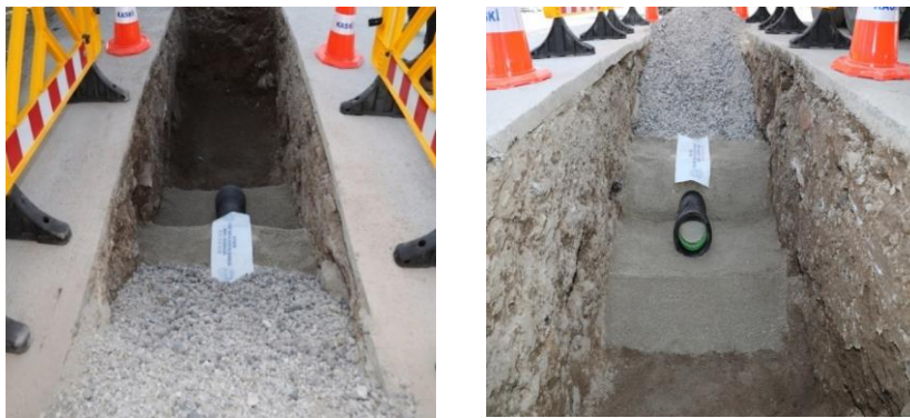
Figure 1. Network renewal in the field
