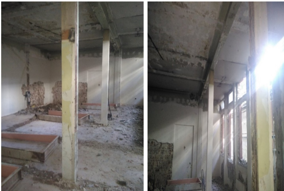
Figure 10. Steel columns and beams added to the building
