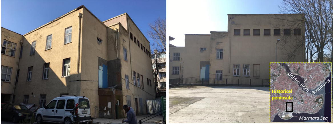
Figure 1. The current condition of the examined building
