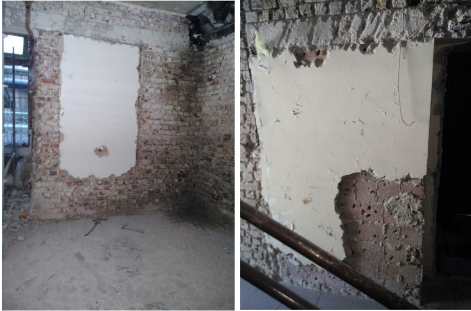
Figure 9. An opening cut in the masonry wall (later closed)
