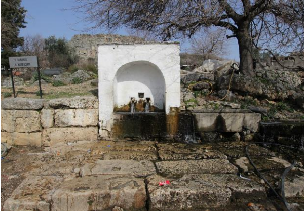
Fig. 16. Kocagözler Fountain, a general view from west
