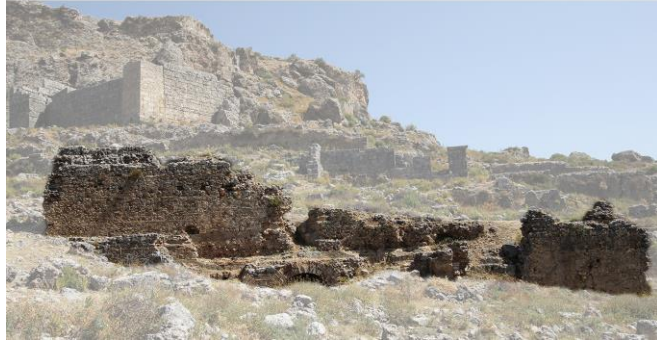
Fig. 13. Nymphaion A / Fountain of Late Antiquity, drawing of facade and a general view from west
