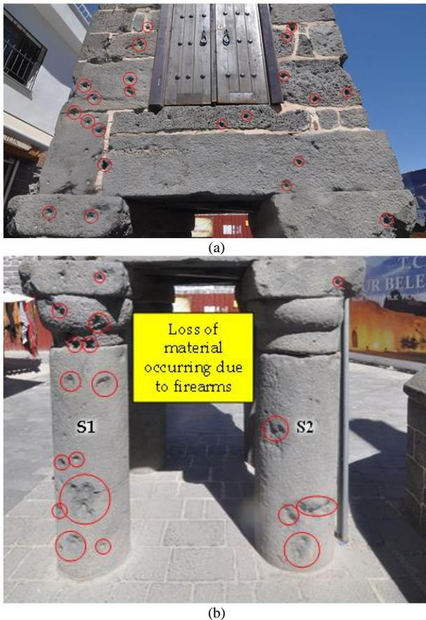
**Figure 10.** Photographic views of damages caused by firearms on: (a) the body and (b) columns of the Four-Legged Minaret (taken in 2021)
