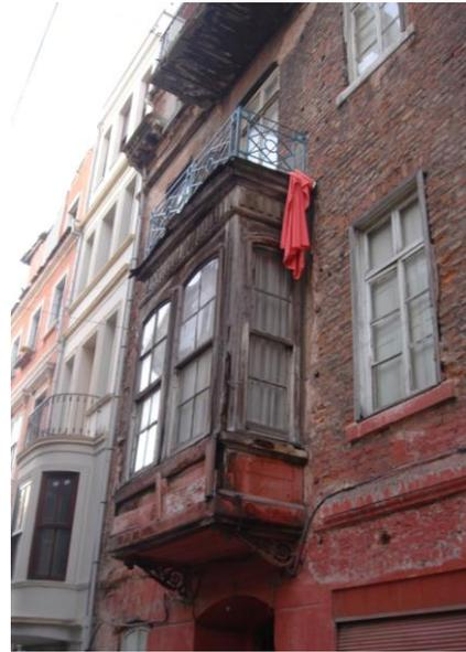
Fig. 10 A timber constructed jetty from a house at Serdar-ı Ekrem street, Galata (Photo: B. S. Coşkun 2015)
