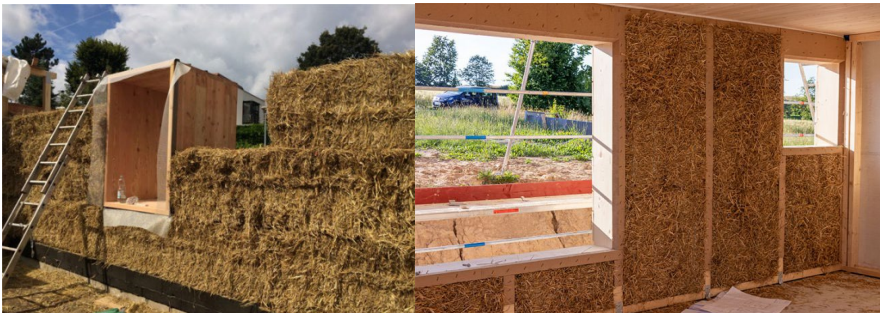
Figure 4: Load-bearing Straw Bale Wall (left). Photo Z Architektur (Fromm, 2022), and infill Straw Bale Wall (right). Photo Bruno Mader (Jeske, 2021).
