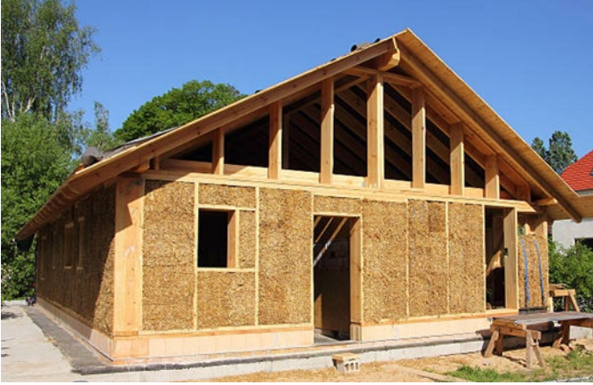
Figure 6. House of Straw. Constructed with infill method (qtd. Gallagher, 2022).
