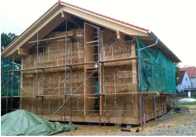
Figure 3: Load-bearing Straw Bale House Construction. Photo Virko Kade (Fromm, 2022).
