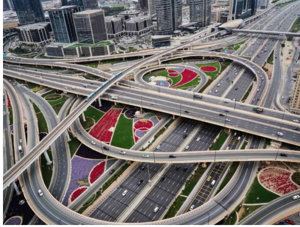
Figure 19. Dubai Streets as the example for pipes [40].
