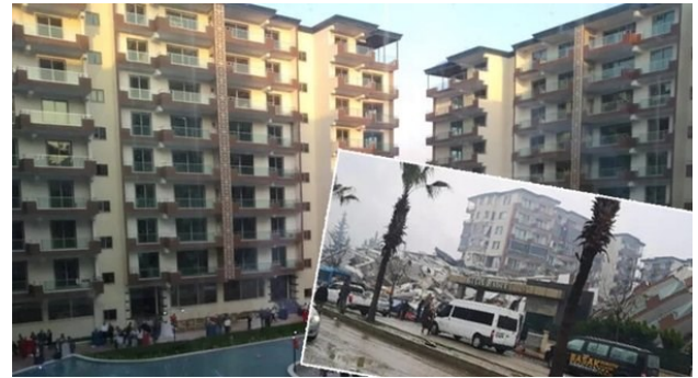
Figure 19. A nine-storey building in Antakya
