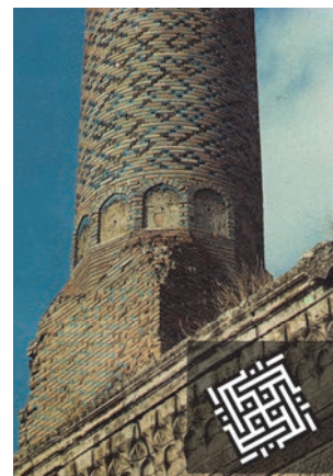
Figure 50. Ince Minareli Medrese, Konya of 1258, square kufi cut-tile mosaic, the Word, Muhammad. Inset Square kufi Muhammed repeated 4 times in a square.
