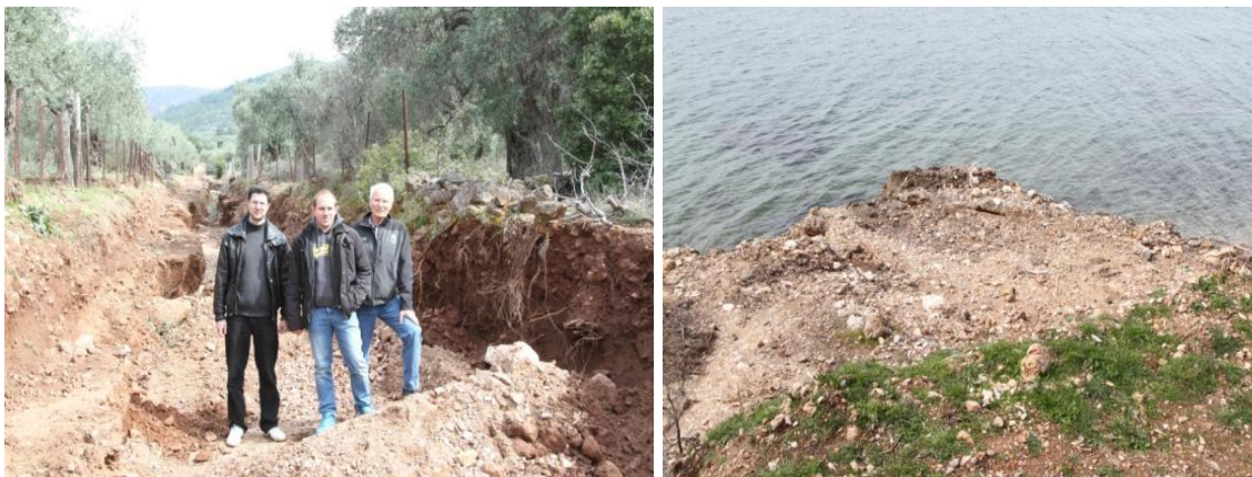
Figure 2. The severe wildfire in Kalirahi watershed of Thasos Island in August of 2013 led to severe surface runoff events in the spring of 2015. This led to the wash out of this gravel road in Kalirahi watershed in Thasos Island by the excessive runoff the led to erosion (left). The eroded material were deposited along the seacoast and in the sea (right).
